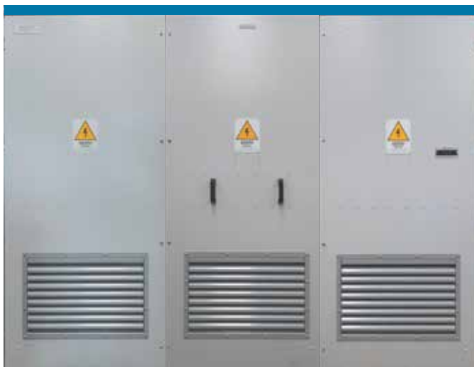
INCOMING LINE AND MAIN TRANSFORMER SECTION
